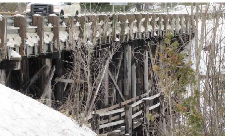
bove is Doug Field's photo of the wonderful 66 Year old bridge, crossing Eels Creek on Highway 28 at Haultain, which is one of the final few remaining wooden bridges in Ontario supporting a major highway. It was built in 1952 and the Apsley Voice has learned that it will soon be replaced with a new, two lane, single-span, steel girder bridge set to last 75 years.
